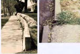
Left: Creeping along the Calaveras fault has bent the retaining wall and offset the sidewalk along 5th Street in Hollister, California (about 75 km south-southeast of San Jose). Right: Close-up of the offset of the curb. (Photographs by W. Jacquelyne Kioua.)
